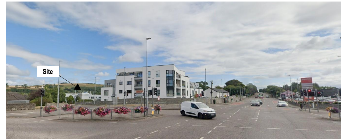
Existing View from the City West Mews Road looking East.
